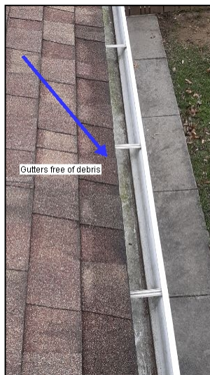
Gutters were clean and free of debris.
