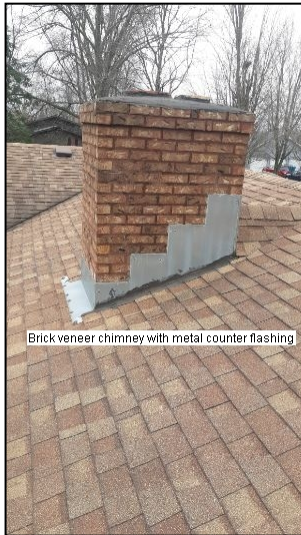
Brick veneer chimney is good condition and was properly flashed.
